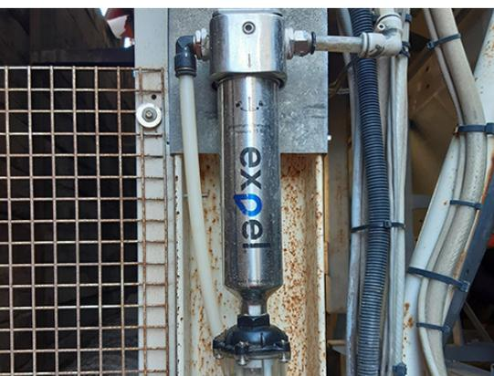
AVG EXPEL Compressed Air Filter installed
