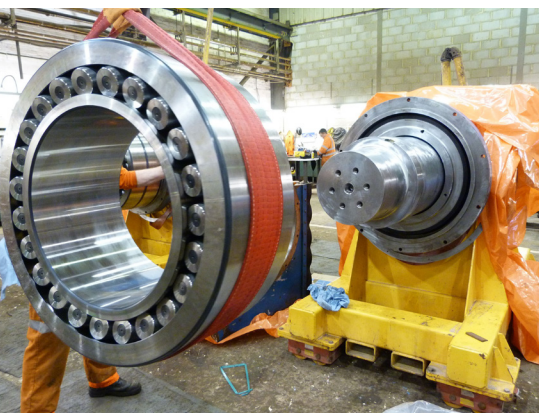
Mounting the bearing onto the shaft
