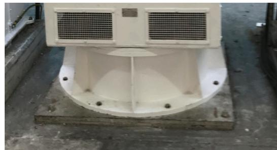
Excessive vibration due to loose flange bolt. 1/2 turn achieved on rear bolts, 2 full turns on front bolts
